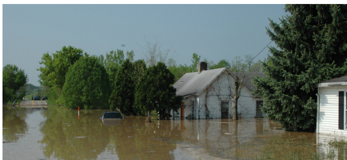
Red Cross volunteers assess flood damage in Ross County, Ohio.
